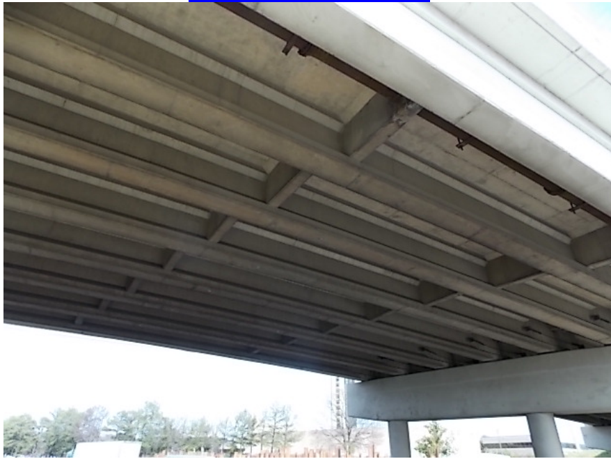
BOTTOM DECK SPAN 3
